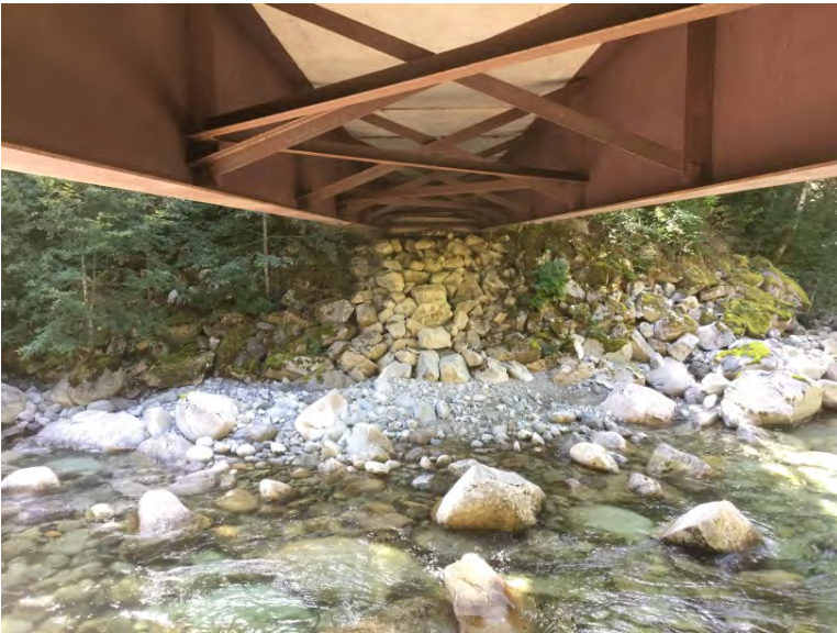
Right Bank Abutment when facing downstream
