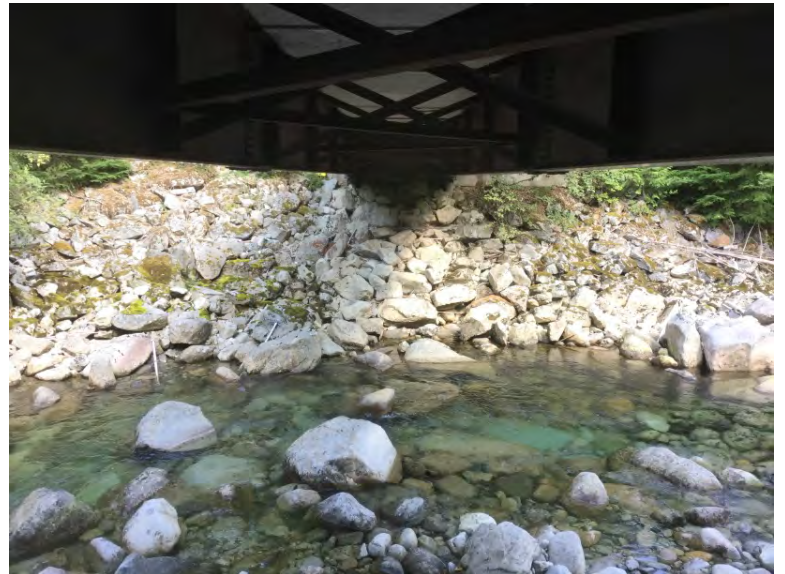
Left Bank Abutment when facing downstream
